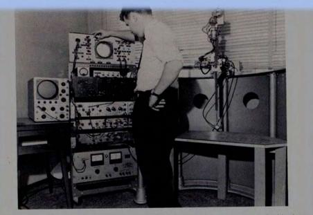
Figure 11. An abdominal echoscope constructed in 1962 by G. Kossoff, who is seen in this picture. The transducer is attached to the rack on the right of the photograph, and in clinical use it is immersed in a water tank; the patient is positioned with her back supported by an inclined couch, with her anterior abdominal wall in contact with a flexible membrane that forms one of the walls of the water tank.
